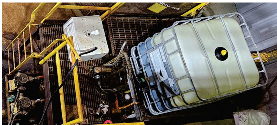
Photo 53: Ferric Chloride Pumps (2) and Tote
