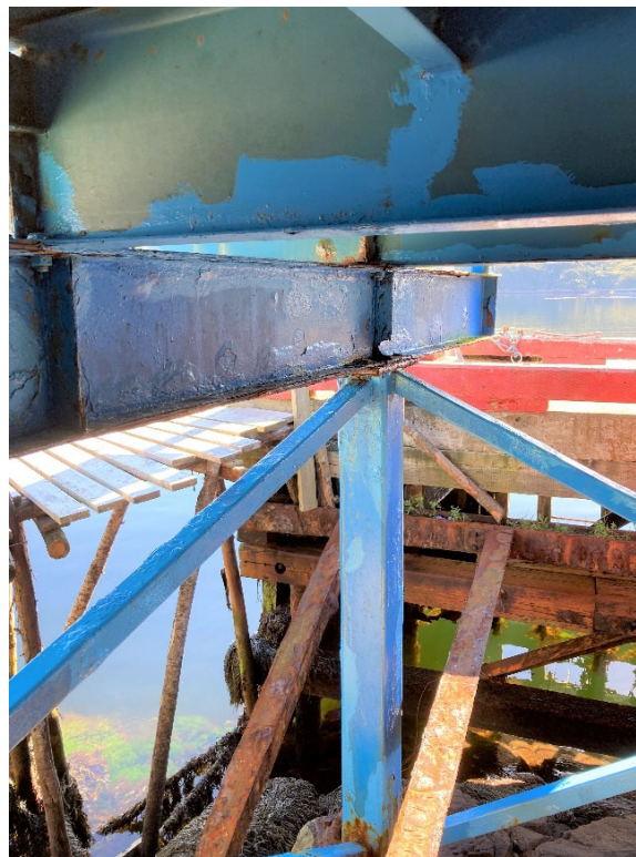
Photo 4: View at underside of tank – existing beams, column, and bracing members
