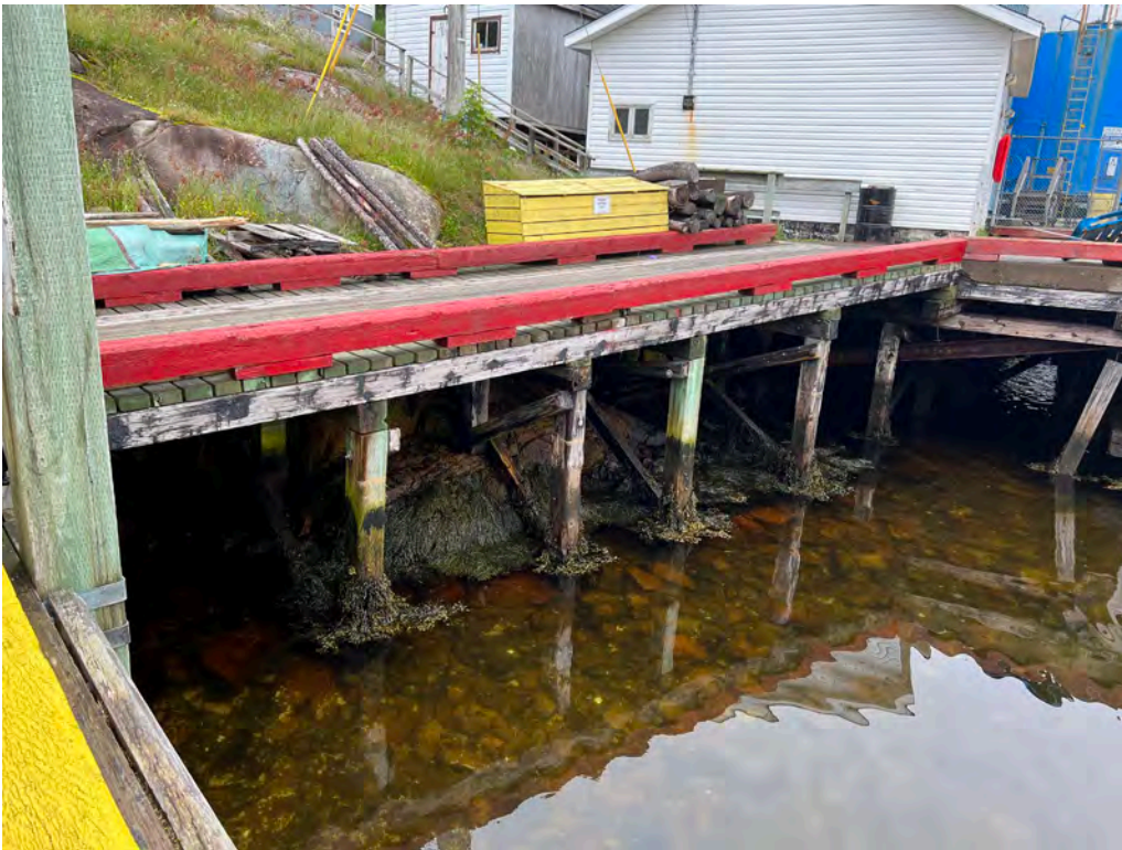
General view showing approach walkway
