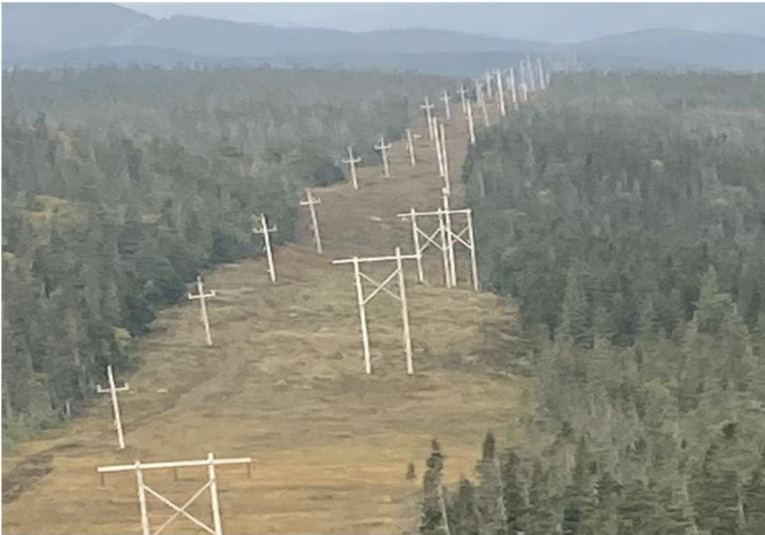
Figure 2: Narrowing of the ROW at the Southern Park Boundary
