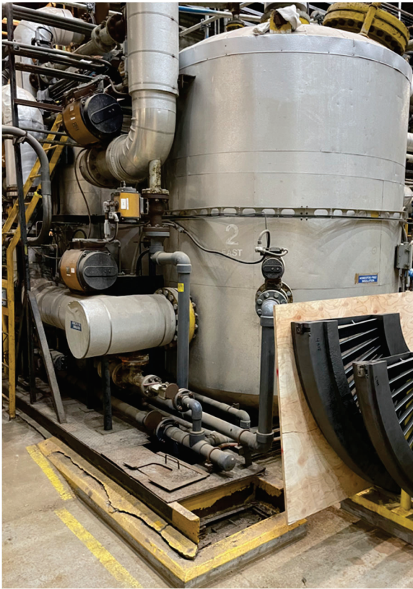
Photos 37 & 38: Unit 2 Condensate Polishers (see deteriorating supports)
