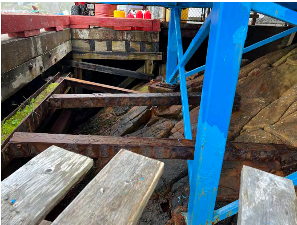
Tie-back angled bracing behind piles 1B and 2B
