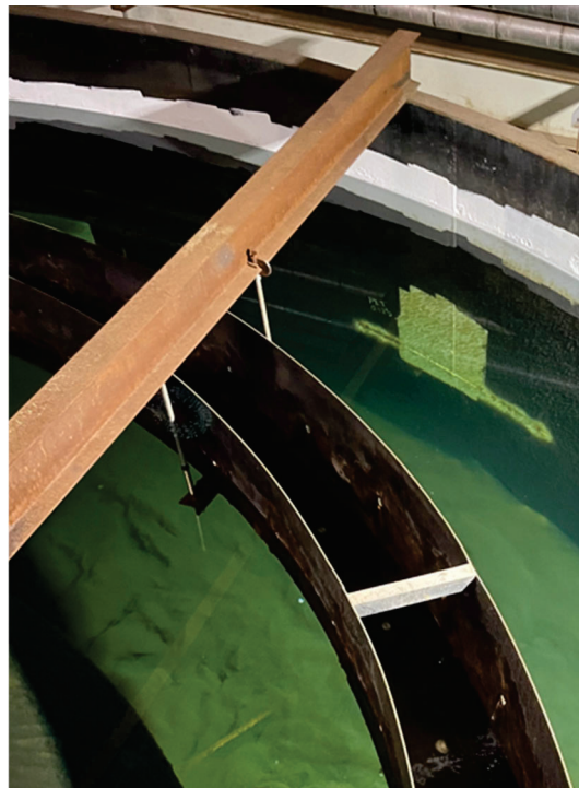
Photo 3: Walkway Structural Support and Trough
