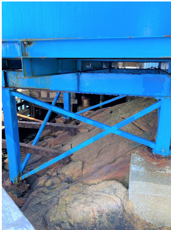
Photo 10: View of beams, columns, and bracing members for the support structure
