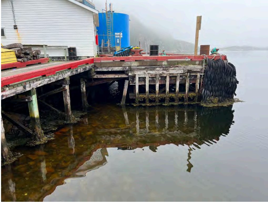
General view showing west end of wharf
