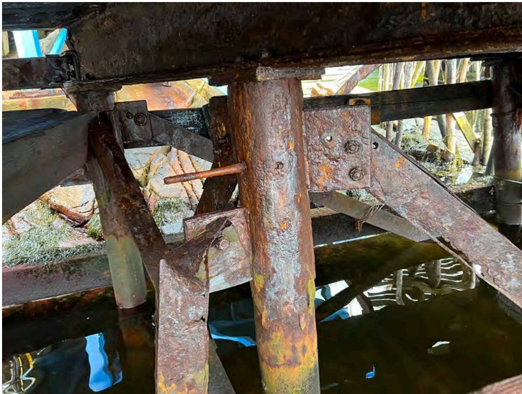
Piles, bracing and pile cap (typical)
