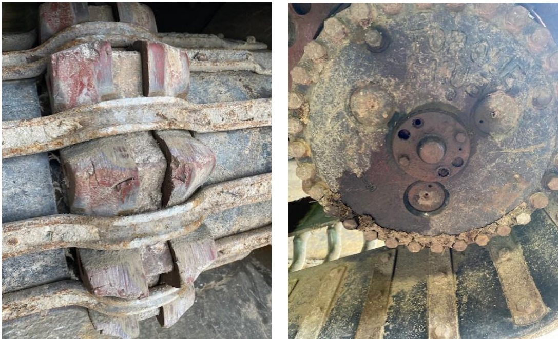
Figure 5: V7698 Final Drive and Sprocket Condition
