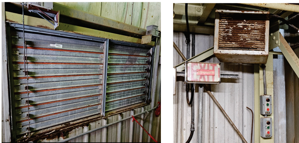
Photos 63 & 64: Existing Air Intake Louvre and Typical Unit Heater
