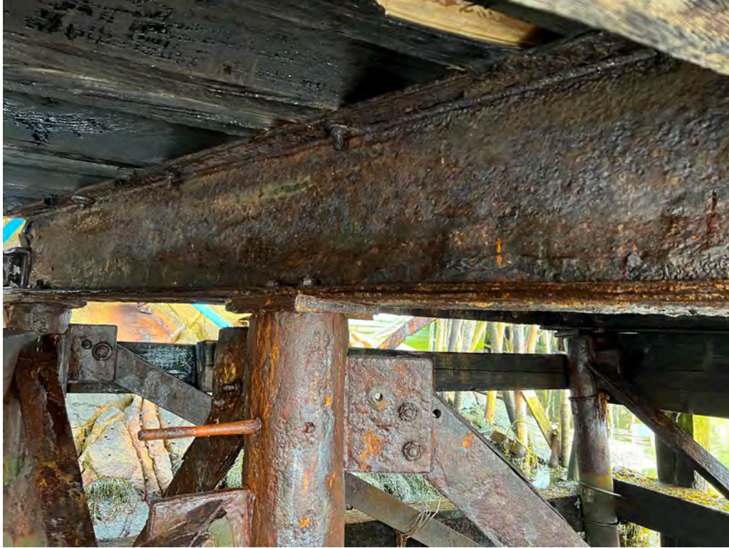
Piles, bracing and pile cap (typical)
