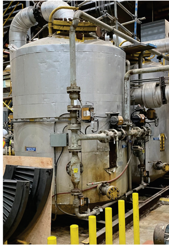
Photos 37 & 38: Unit 2 Condensate Polishers (see deteriorating supports)
