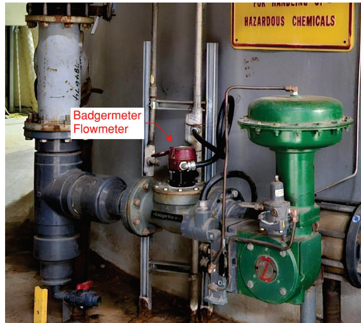
Photos 2A & 2B: Clarifier Piping and Badgermeter Flowmeter.
