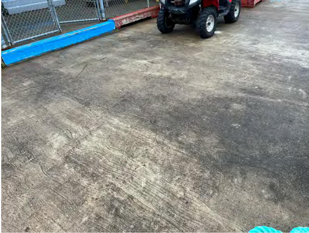
Concrete deck surface
