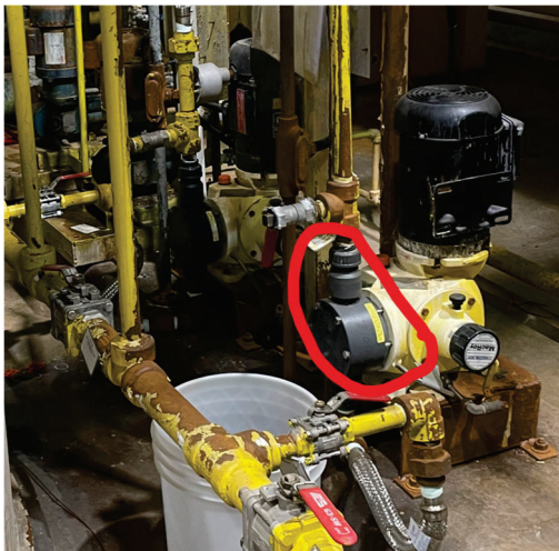
Photos 31 & 32: Acid Transfer Pumps (2)
