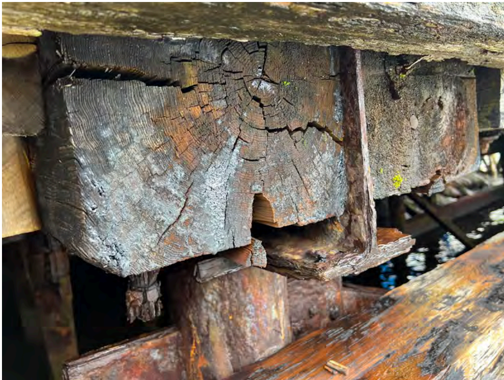
Caps with timber blocking on either side of web
