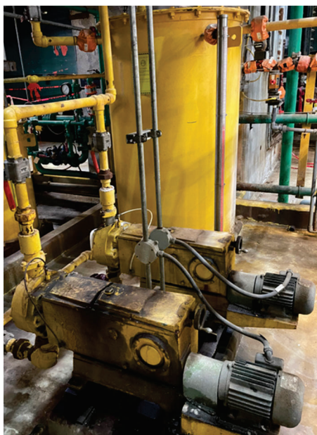
Photo 35A & 35B: Unit 1 Caustic Transfer Pumps and Day Tank (left) and Acid Transfer Pumps and Day Tank (right)
