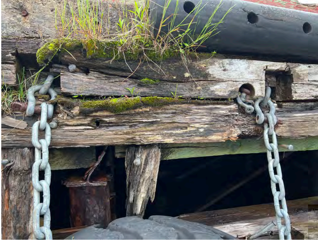
Horizontal rubber fender, chocks and chains for rubber tire fenders
