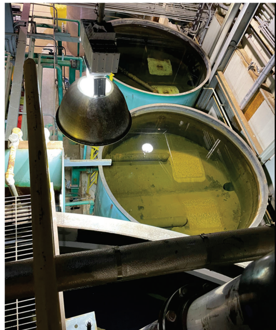
Photo 4B – Plan View of Sand Filters #1 & #2
