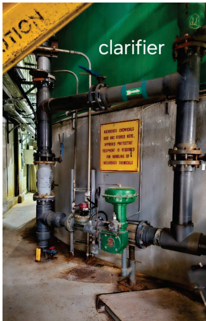
Photos 2A & 2B: Clarifier Piping and Badgermeter Flowmeter.
