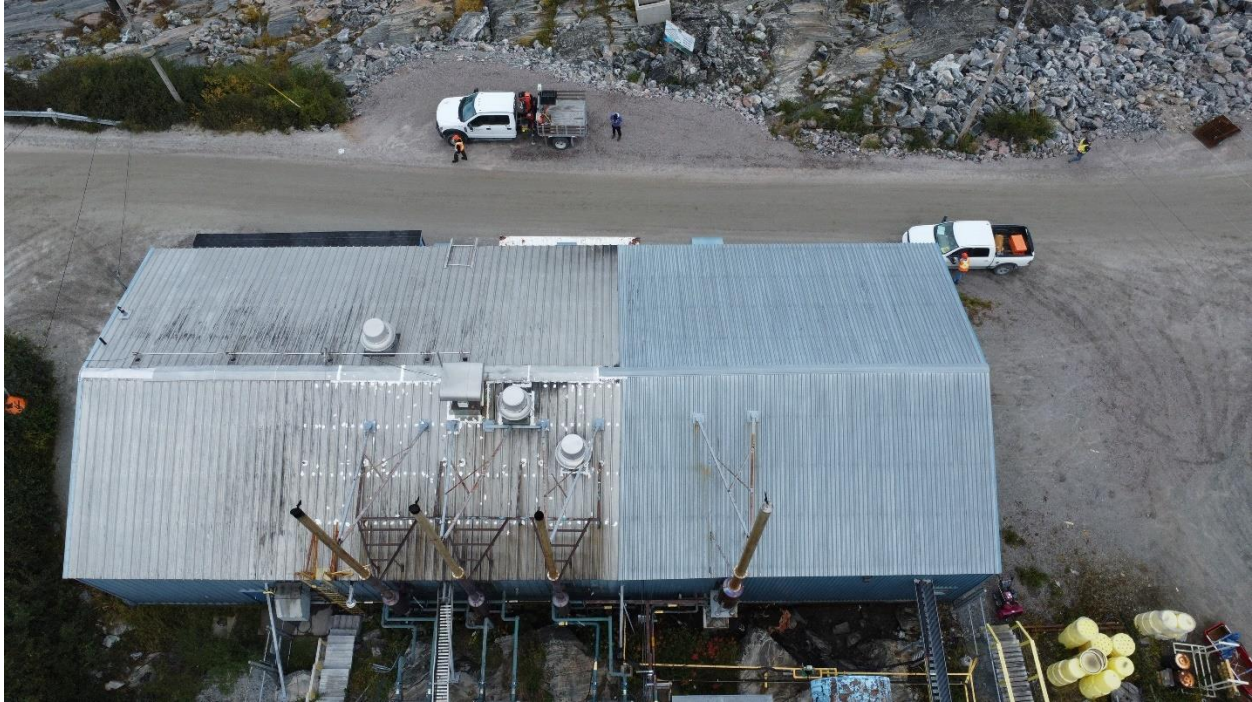
Figure 1: Hopedale Diesel Generating Station Roof
