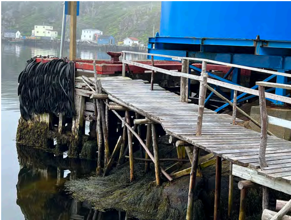
General view showing east end of wharf
