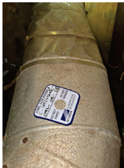
Photos 50 & 51: Caustic Piping (Utilidor)
