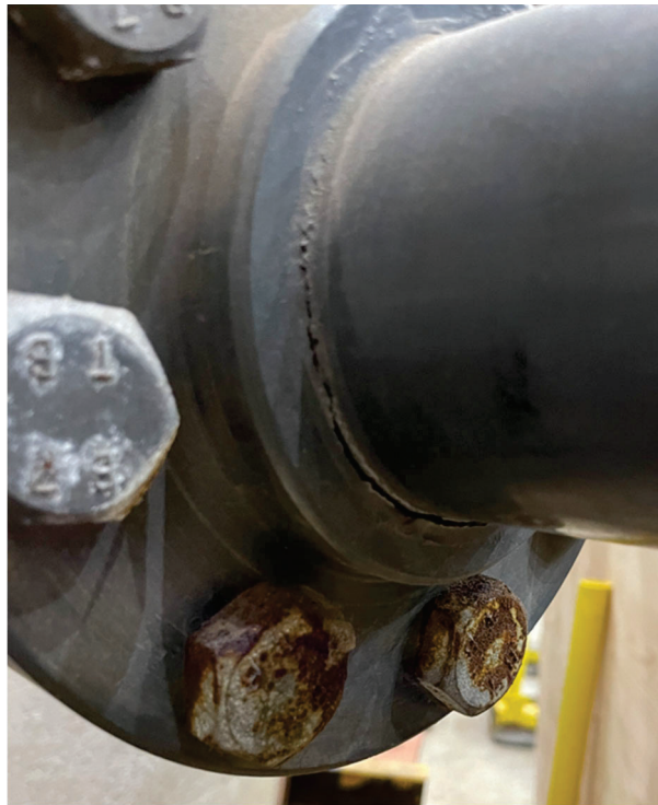
Photos 39A & 39B: Unit 2 Piping Starting to Separate due to Polishers Dropping
