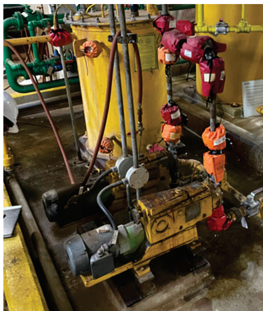
Photo 35A & 35B: Unit 1 Caustic Transfer Pumps and Day Tank (left) and Acid Transfer Pumps and Day Tank (right)
