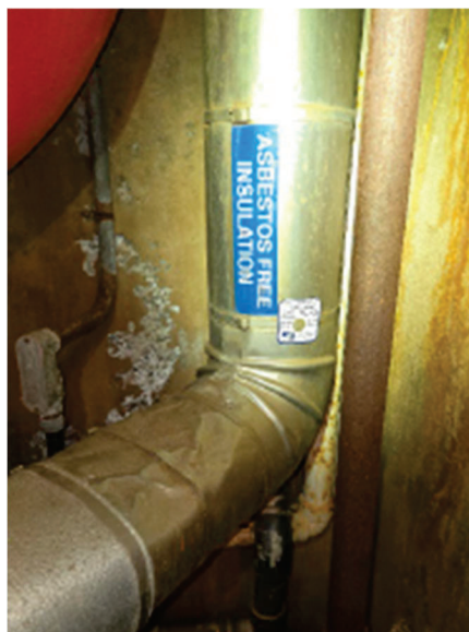
Photos 50 & 51: Caustic Piping (Utilidor)
