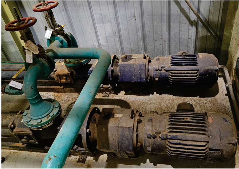
Photo 56: Sludge Pumps
