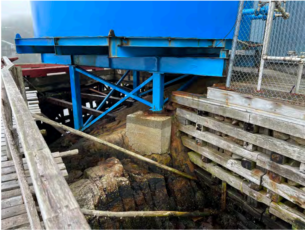
Elevated tank on east end behind Row "B" of wharf
