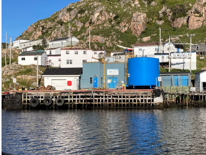
Photo 1: View of existing tank located behind the wharf
