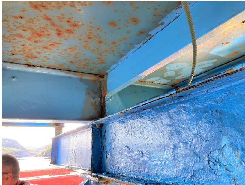
Photo 2: View of main support beam
