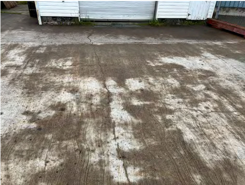
Concrete deck surface
