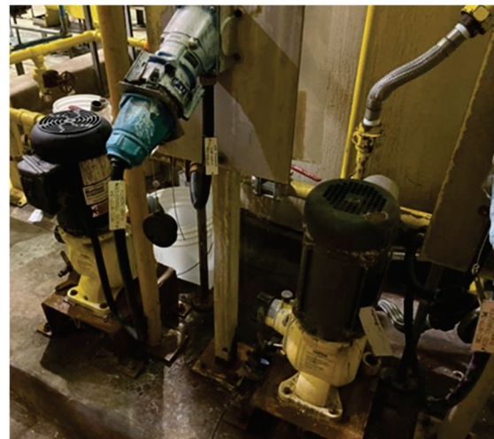
Photos 31 & 32: Acid Transfer Pumps (2)
