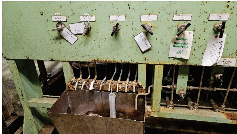
Photos 34D, 34E & 34F: Unit 1 Sampling Station and Sodium after Polisher
