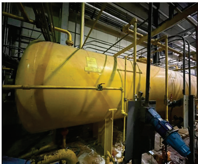
Photos 21 & 22: Caustic Soda Storage Tank and Transfer Pumps
