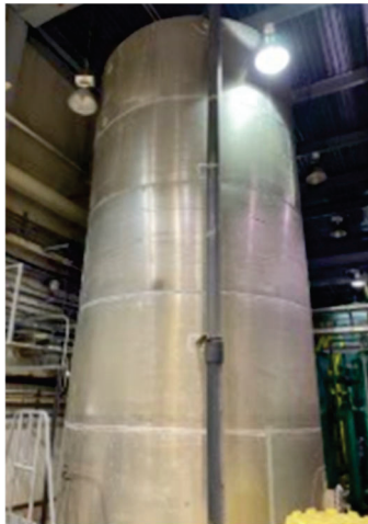
Photo 27: Demineralization Tank
