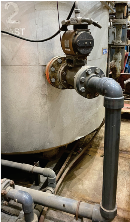
Photos 39A & 39B: Unit 2 Piping Starting to Separate due to Polishers Dropping
