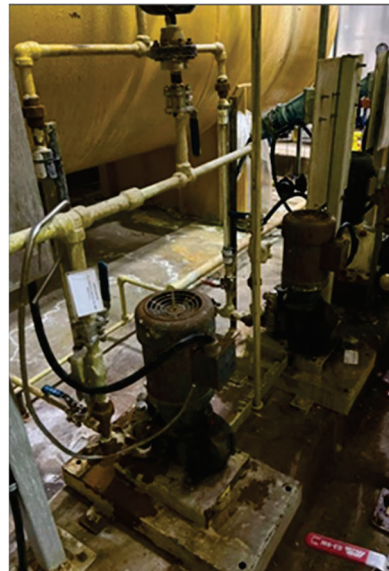
Photos 21 & 22: Caustic Soda Storage Tank and Transfer Pumps
