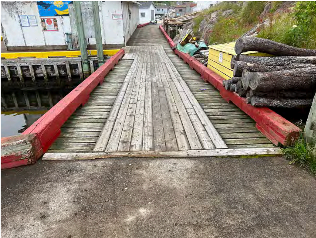
Western walkway approach
