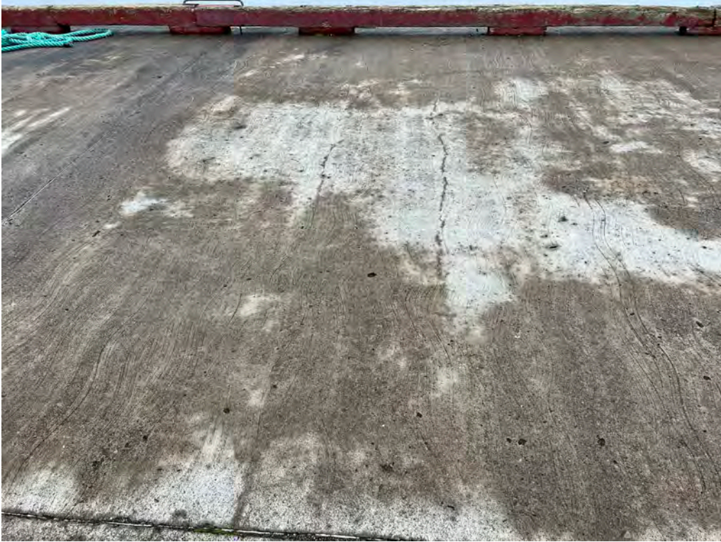
Concrete deck surface
