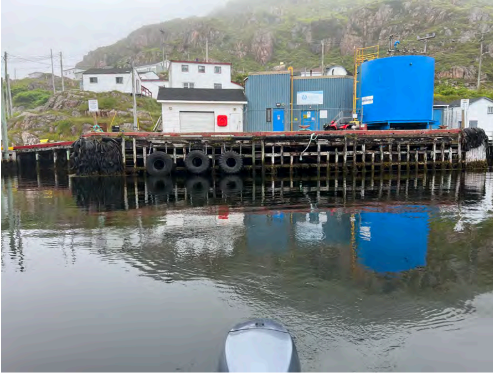
General view showing berthing face
