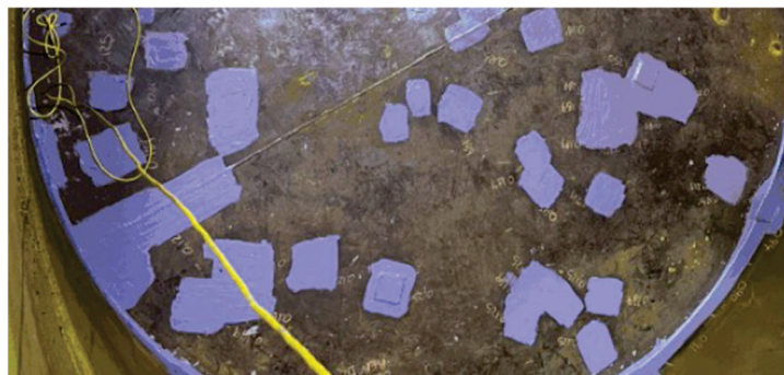
Photo 9: Repairs to Clearwell Bottom
