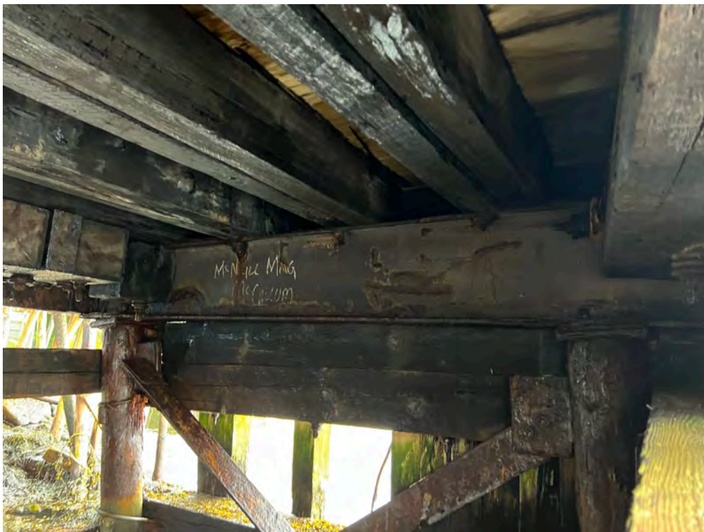
Typical underside showing timber deck beams
