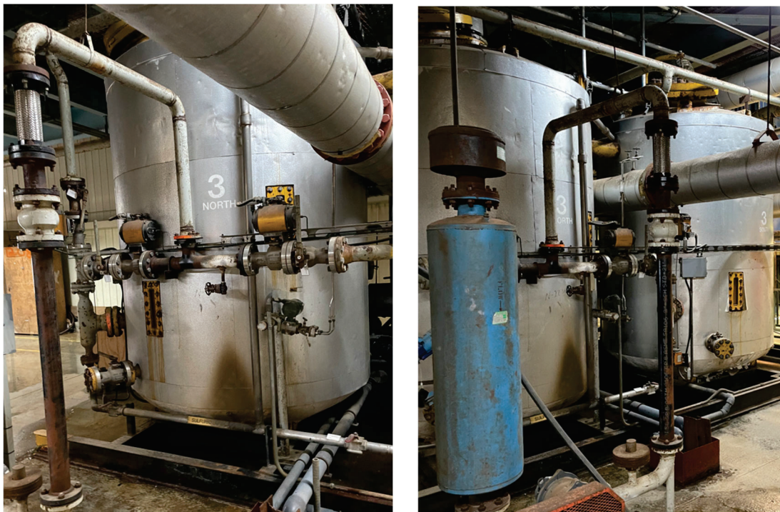
Photos 43A & 43B: Unit 3 Condensate Polishers
